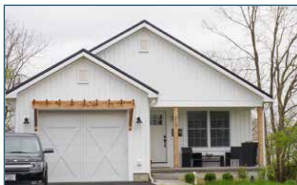
Existing Lebanon housing stock
