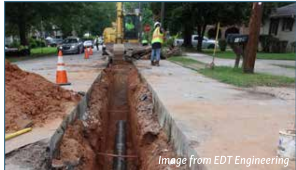
Water main replacement in Atlanta, GA
