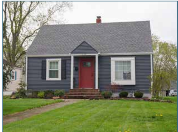
Proactive code enforcement encourages maintenance and upkeep
